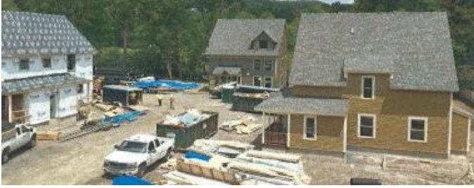
Safford Commons in Woodstock under construction
